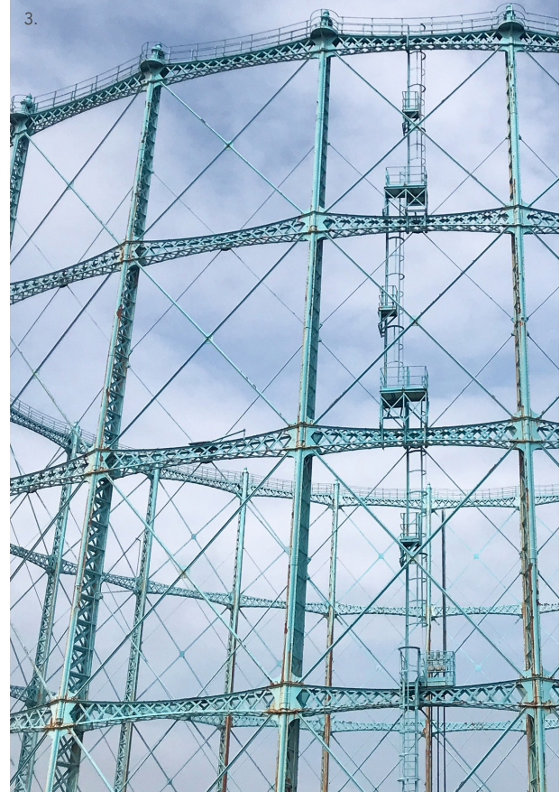
1. Granton Railway Station 2. Former Maldevic Car Factory 3. Granton Gasometer
